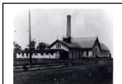
Oshkosh Water Works privately owned by W.G. Maxcy from 1883-1917
