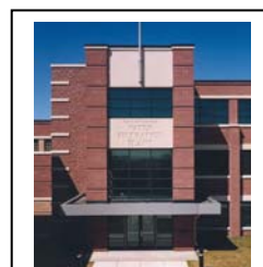
Oshkosh's current state-of-the-art water treatment facility on Lake Winnebago
