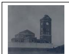
The "new" water filtration plant which was constructed in 1916.
